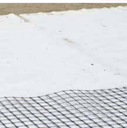
Use of Lotrak® biaxial grid in combination with Lotrak® 200
