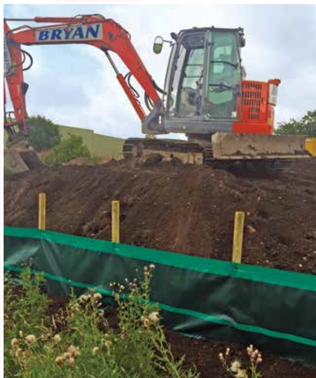
Protection of watercourse using Lotrak® Silt Fence
