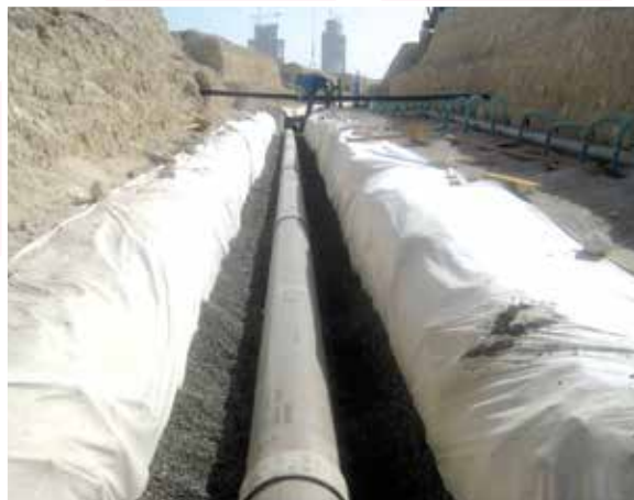
Lotrak® 100 in use in a filter drain
