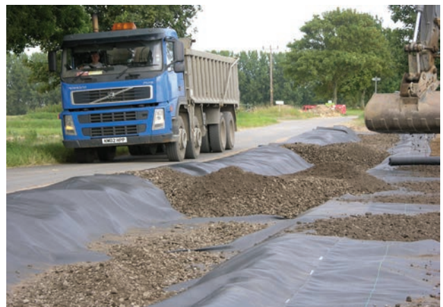
Installation of Lotrak® 50R
