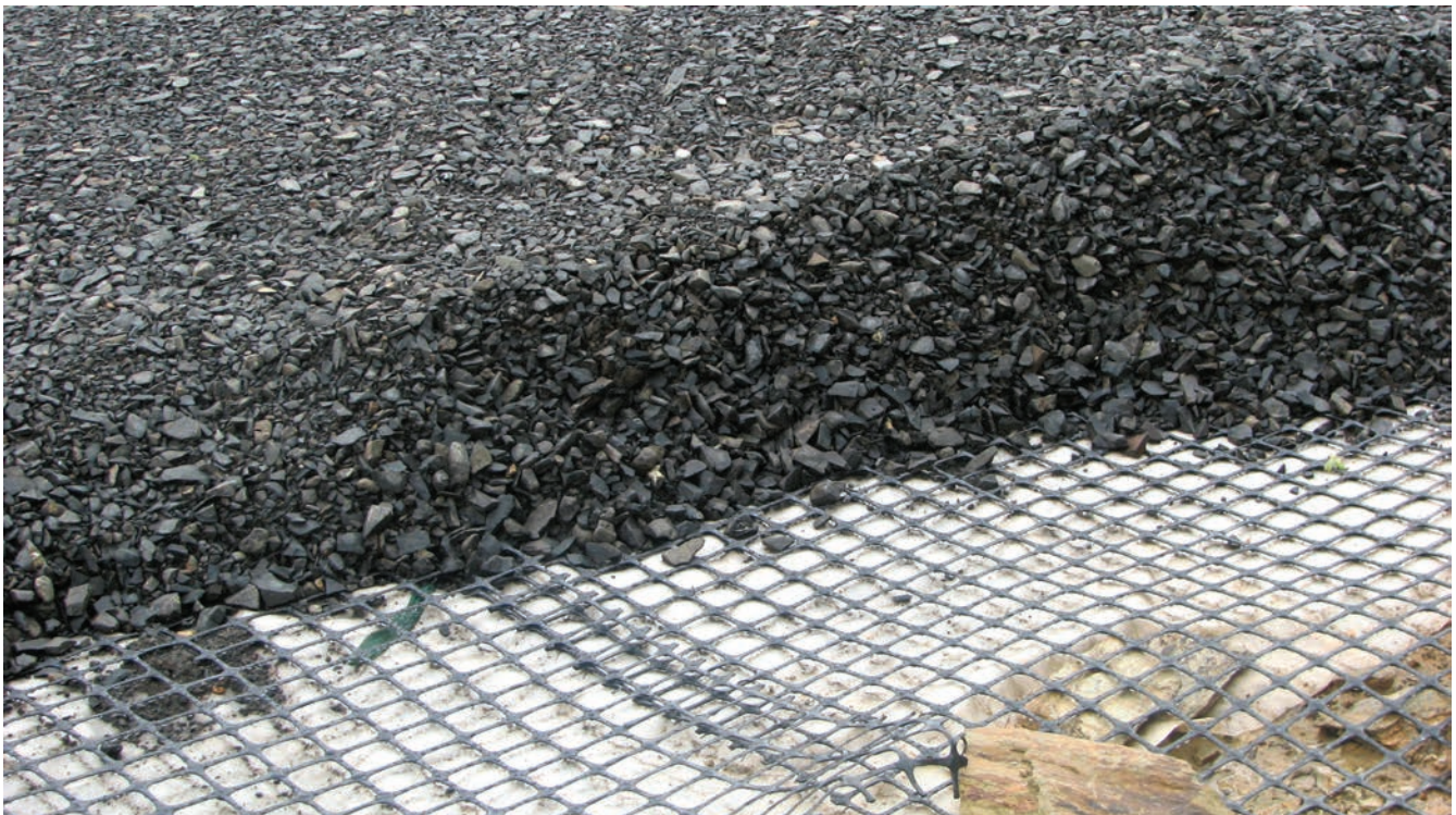
Effective interlock of aggregate material
