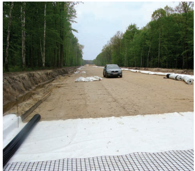
Lotrak® biaxial grid in new road construction
