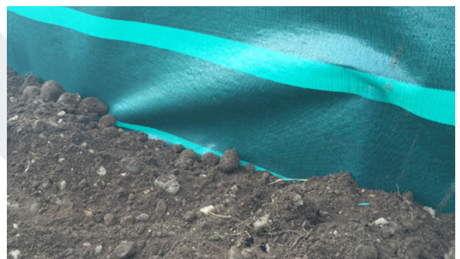
Protection of watercourse using Lotrak ® Silt Fence
